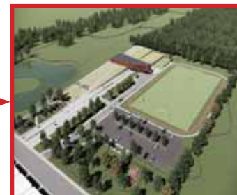
Work-in-progress for the Tamil Community Centre, with the support of Federal, Provincial, Municipal and the Community.
