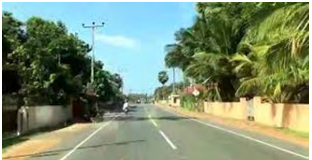
The two ways widened road and parapet walls
