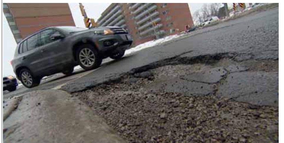
The city tries to get a pothole fixed within four days of it being reported. (Paul Borkwood/CBC)
